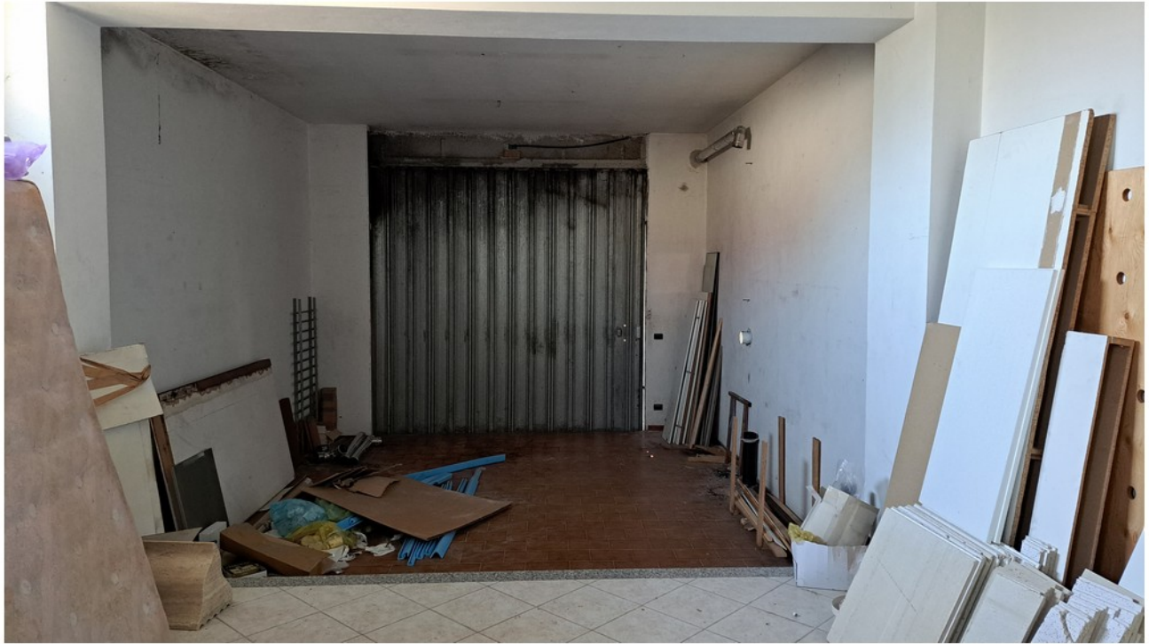
31 - garage deposito piano terra
